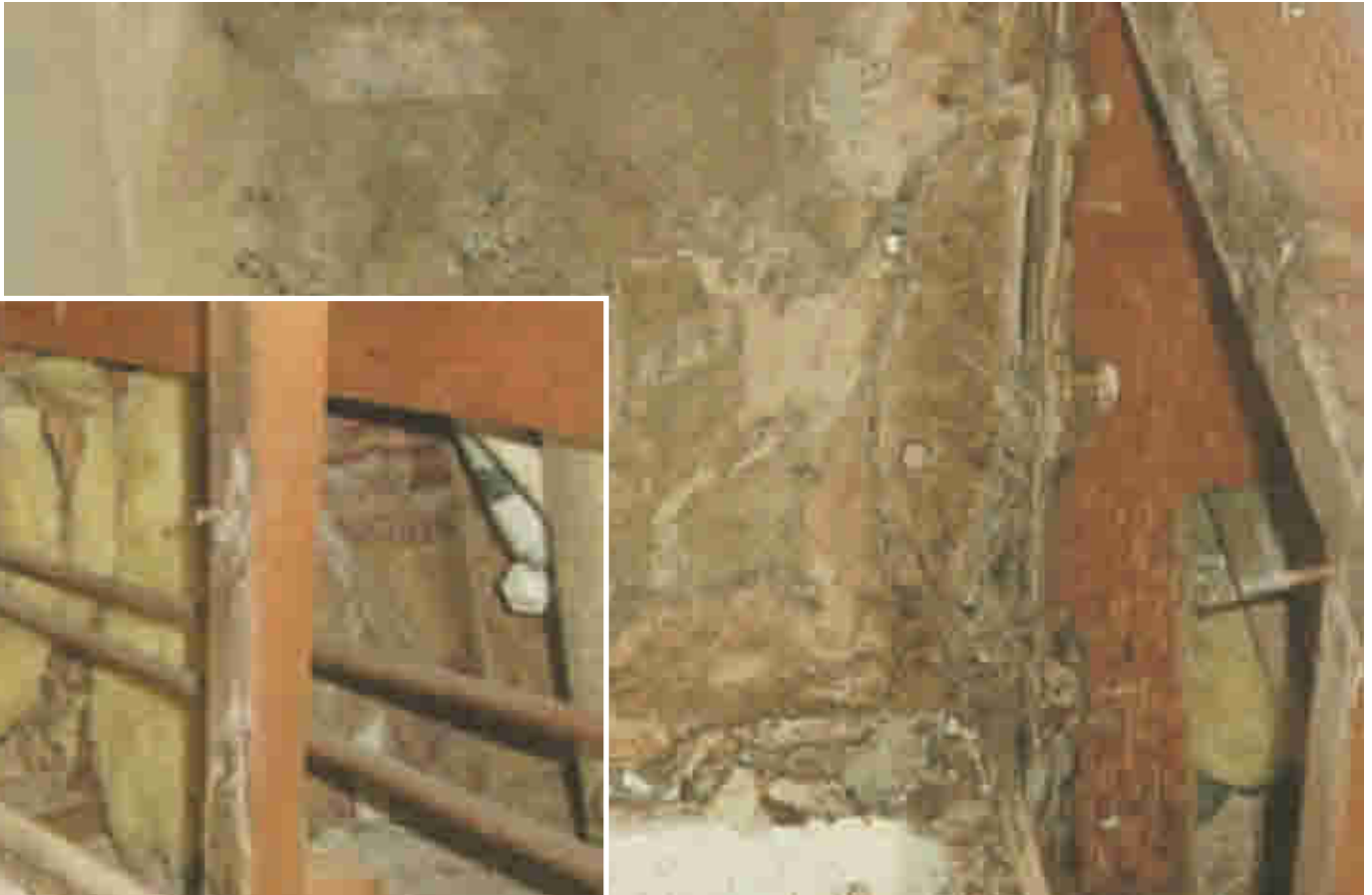
(Below right and left) New wood had to be installed along the pony wall. A light mist of Clorox and water was applied to the entire area to inhibit new mold growth and kill all residual mold.
