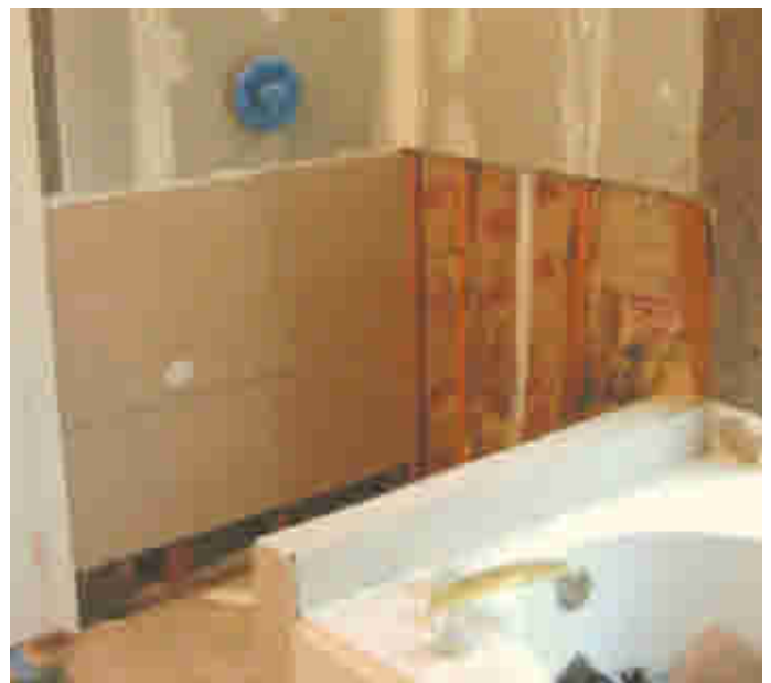
(Below right and left) New wood had to be installed along the pony wall. A light mist of Clorox and water was applied to the entire area to inhibit new mold growth and kill all residual mold.
