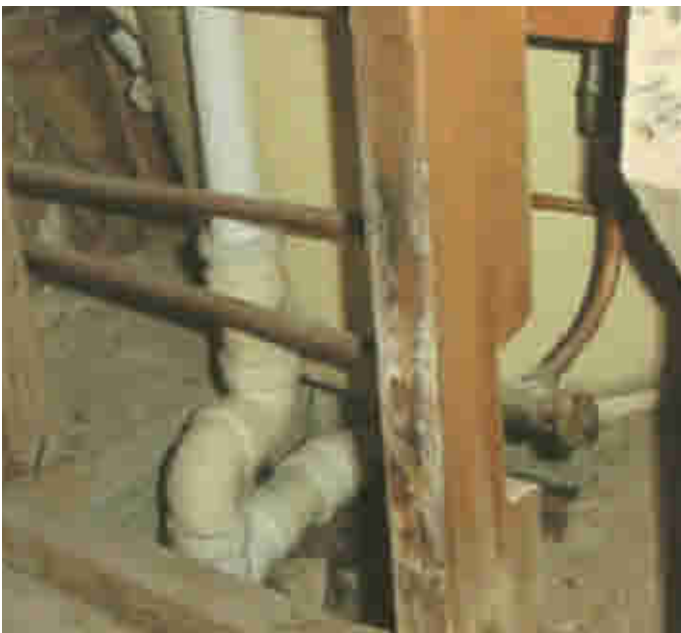
(Above) Additional close up damage mold can cause when moisture wicks behind the shower walls.
