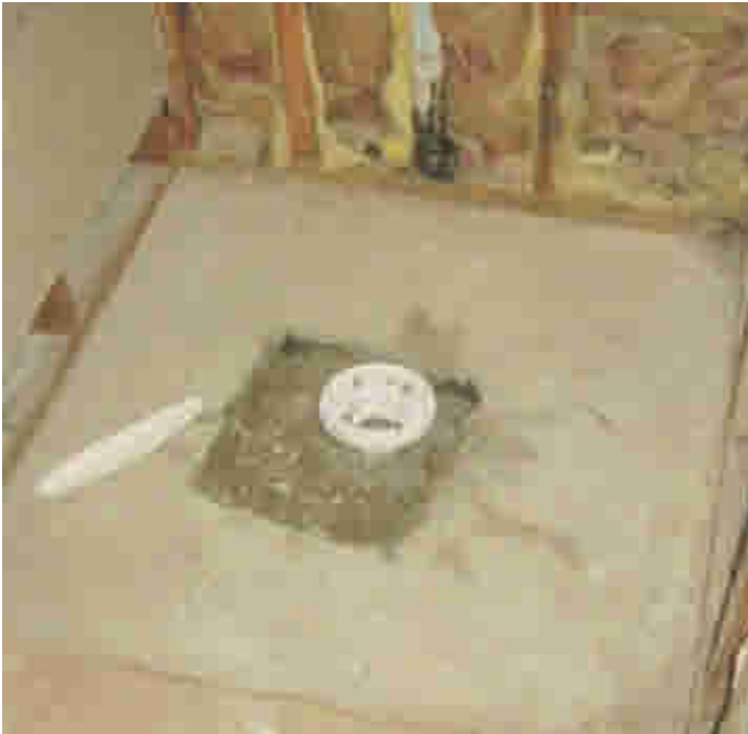
(Above) New FHA drain assembly recessed into the slab.
