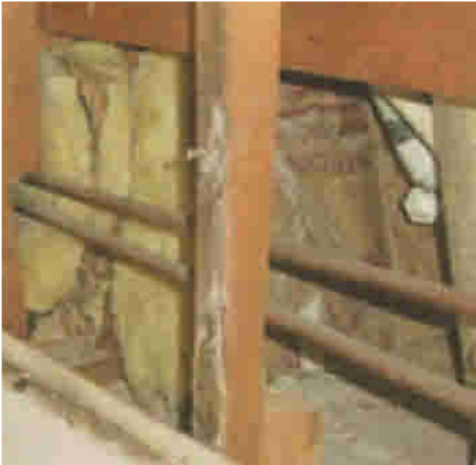
(Above) Additional close up damage mold can cause when moisture wicks behind the shower walls.
